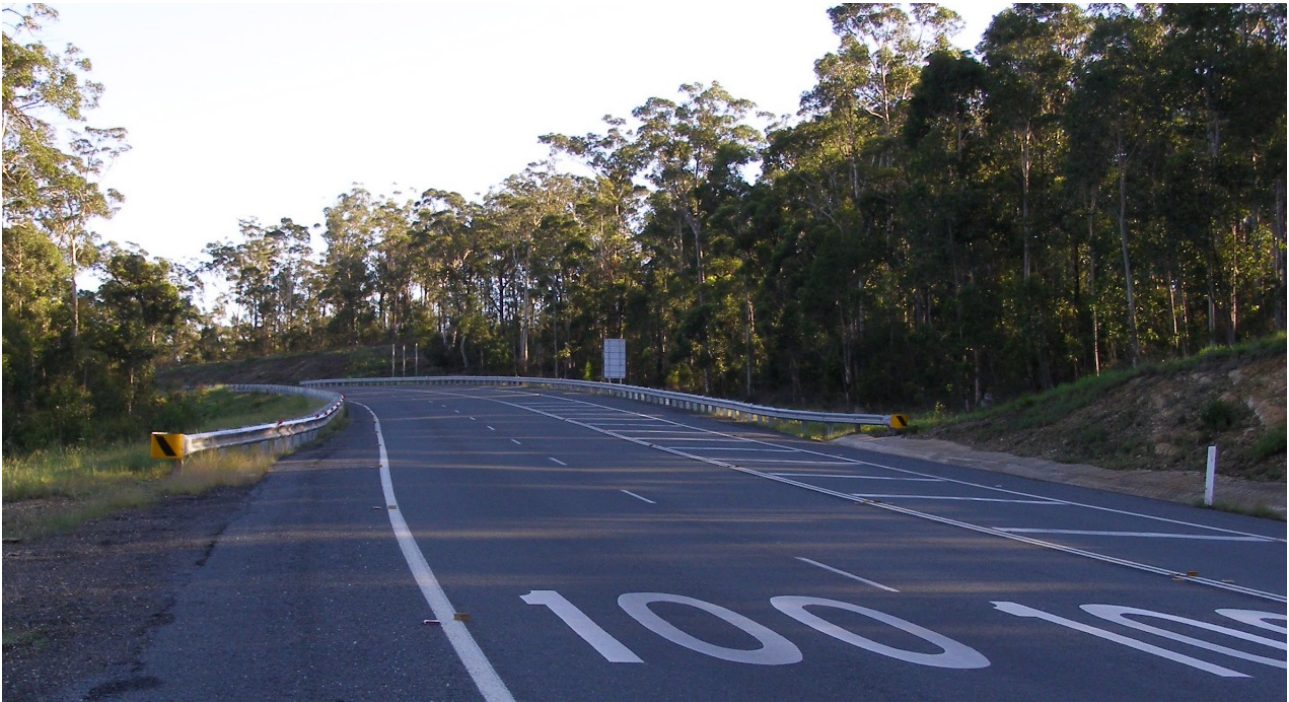
Figure 6.32: Space required for crash attenuators in gore areas
