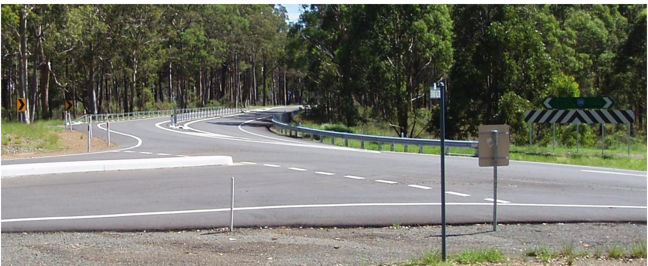
Figure H 1: Wire rope barrier in a narrow median on a sharp bend
