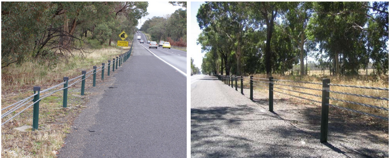
Figure 6.12: Examples of flexible (i.e. wire rope) barrier
