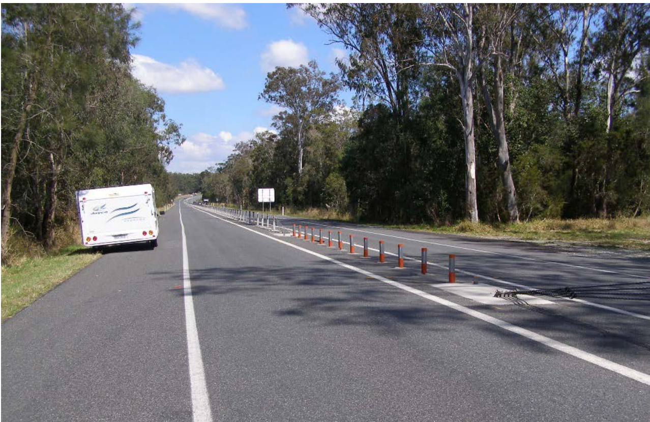
Figure 3.1: Wire rope safety barrier centrally located on a two-lane two-way road
