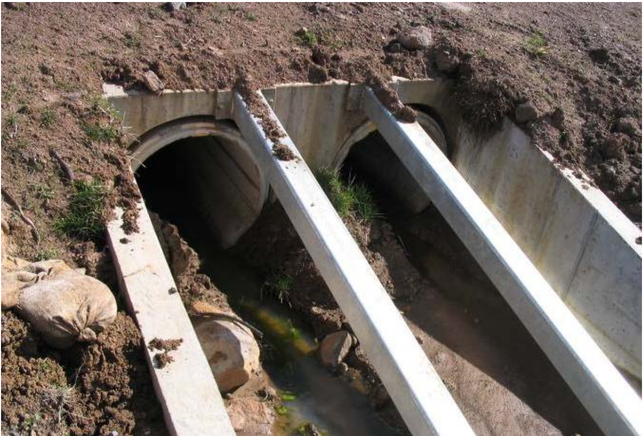
Figure 5.2: Example of a traversable culvert end treatment for a culvert under the road
