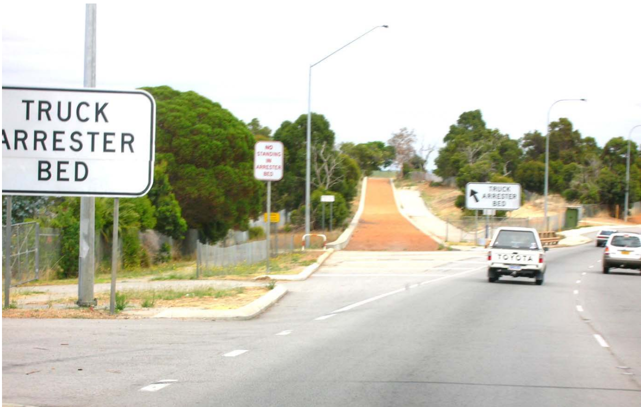
Figure 7.2: An example of an arrester bed
