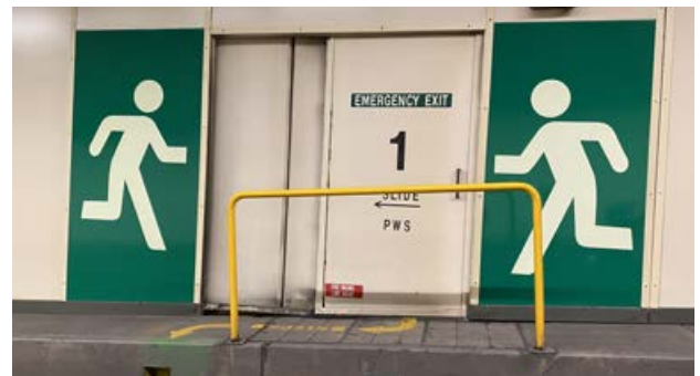
Before and after Sydney Harbour Tunnel emergency exits
