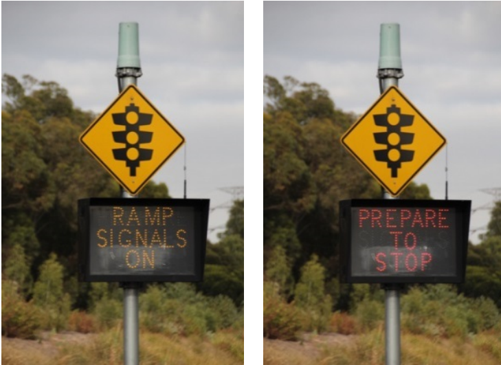
Figure 8.5: Warning signs on entry ramp
