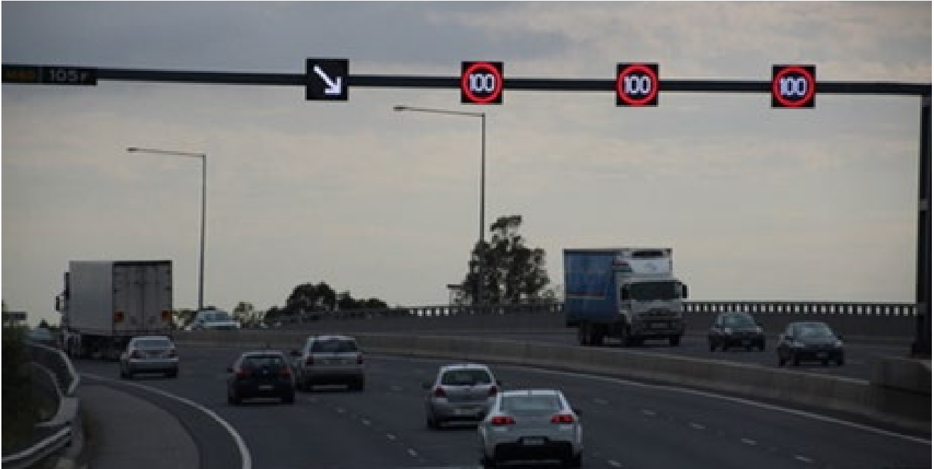
Figure 8.7: Example of LUMS in operation
