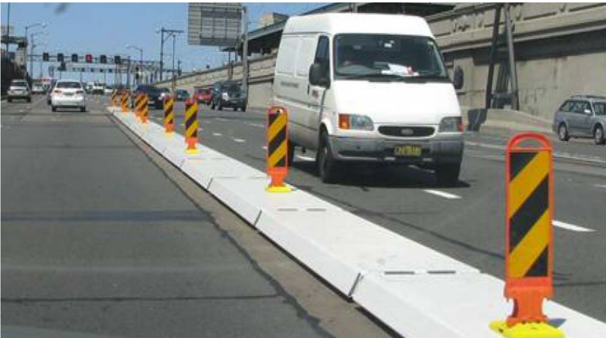
Figure 7.3: Remotely controlled moveable median
