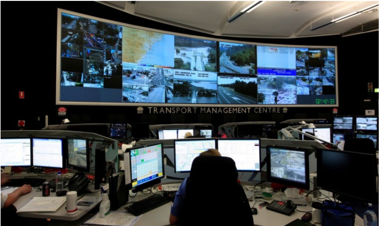
Figure 4.1: Transport Management Centre, Sydney
