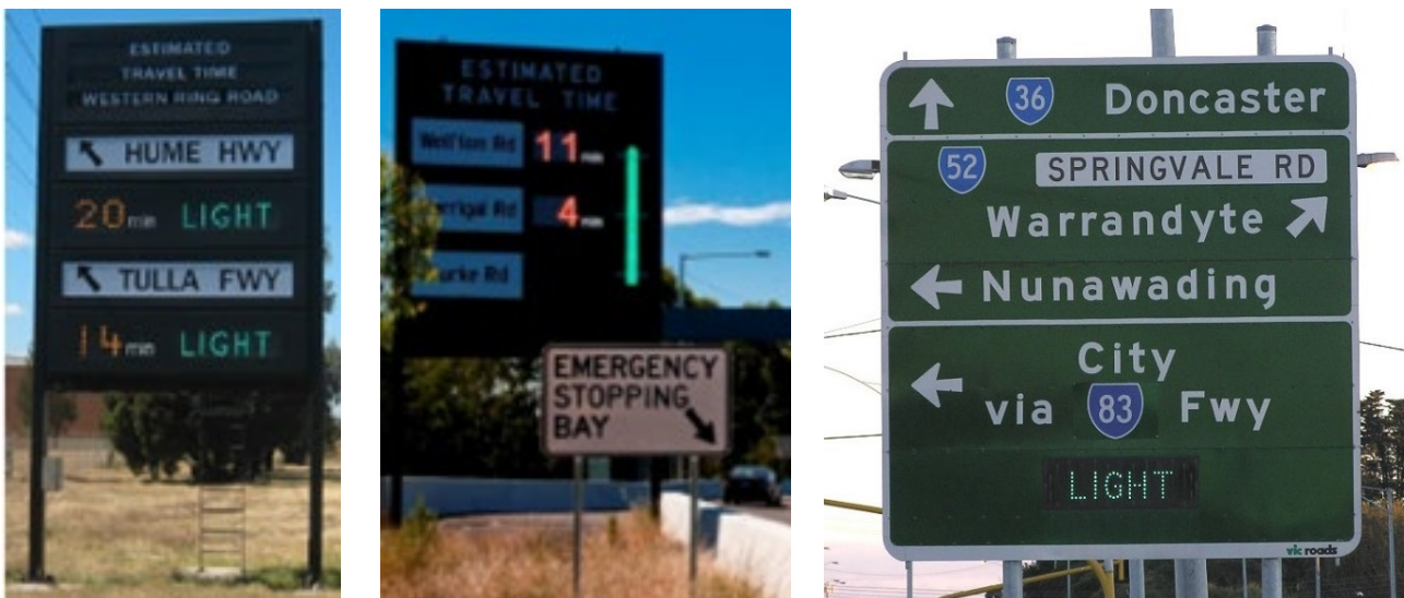
Figure 8.3: Examples of dedicated drive time signs (left and centre) and motorway condition signs (right) in Victoria
