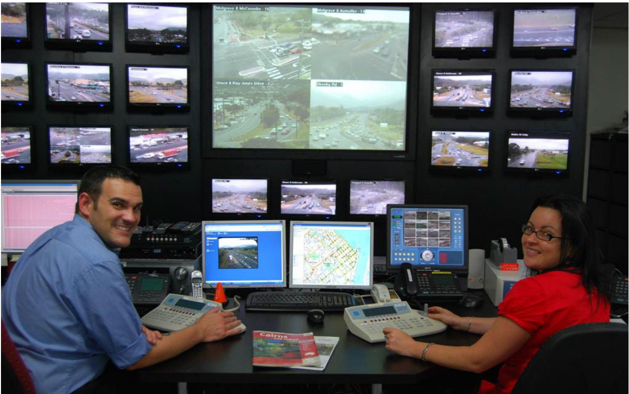
Figure 4.2: Traffic Management Centre, Cairns
