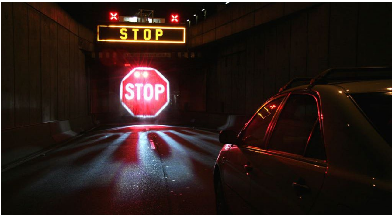
Figure 7.5: Water screen at Sydney Harbour Tunnel
