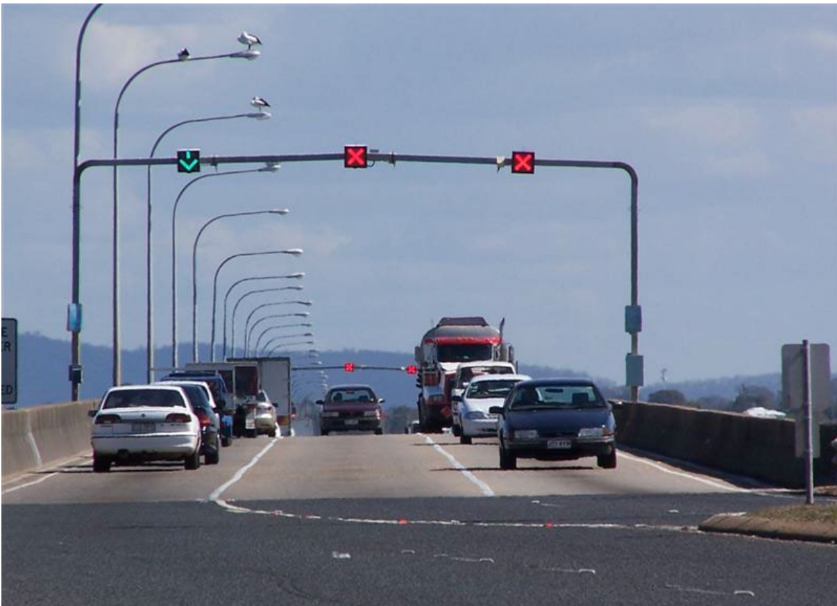
Figure 7.4: Dynamic reversible lane control
