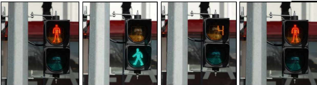
Figure 8.27: Pedestrian traffic signal sequence incorporating the pedestrian countdown timer
