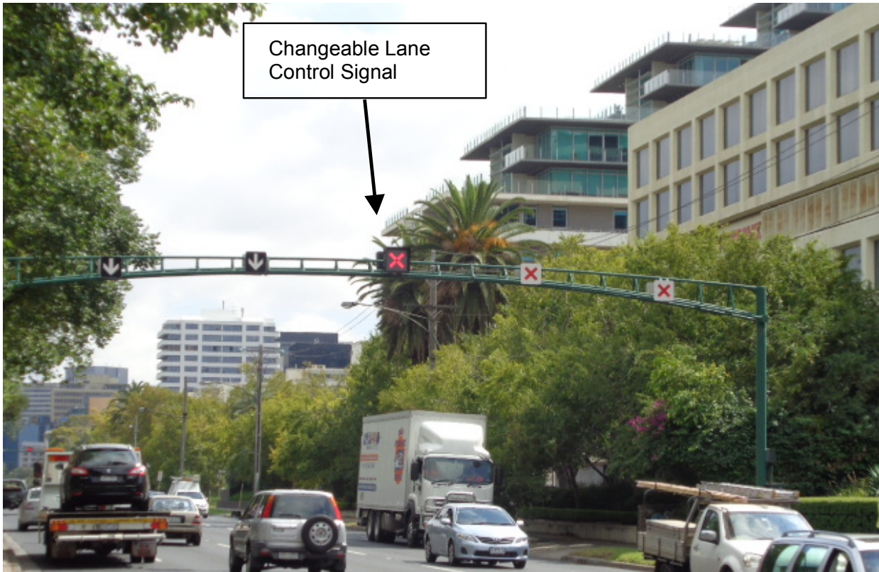
Figure 5.9: Overhead signals for lane reversal
