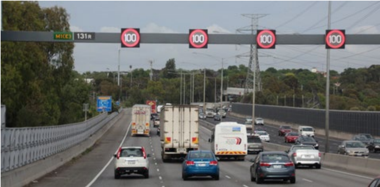
Figure 5.18: ESL above each lane of the carriageway to indicate the limit
