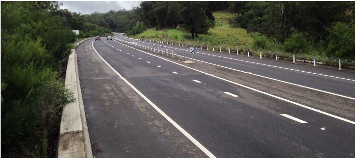
Figure 9.2: Wide centreline treatment with wire rope barrier installed
