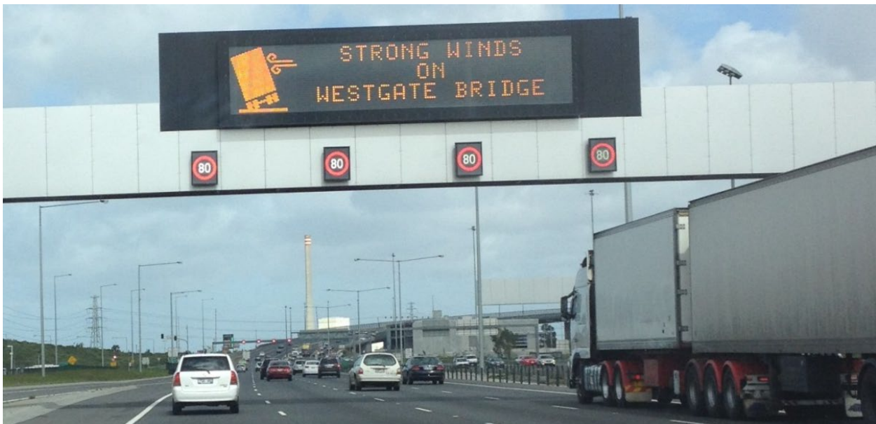
Figure 5.2: Example of a pictogram and text-based VMS
