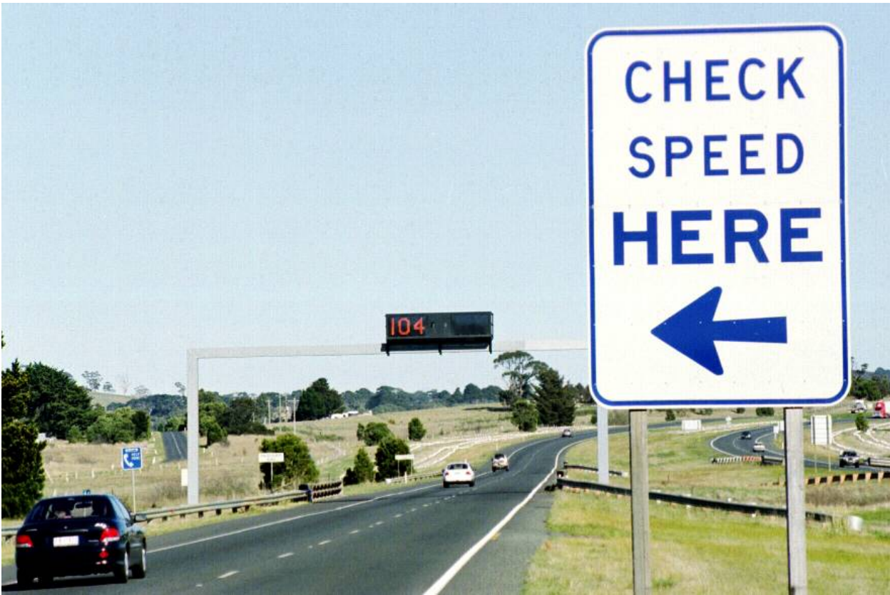
Figure 5.10: Speed indicator system on a motorway
