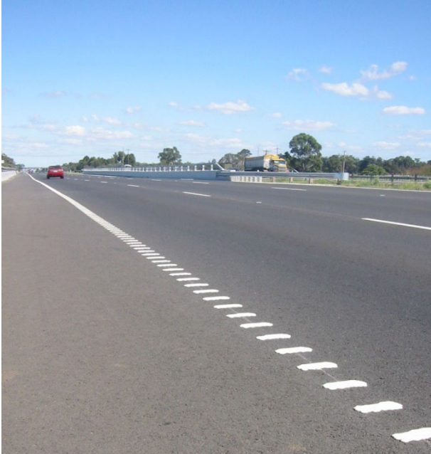
Figure 6.4: Audio-tactile edge lines on a motorway
