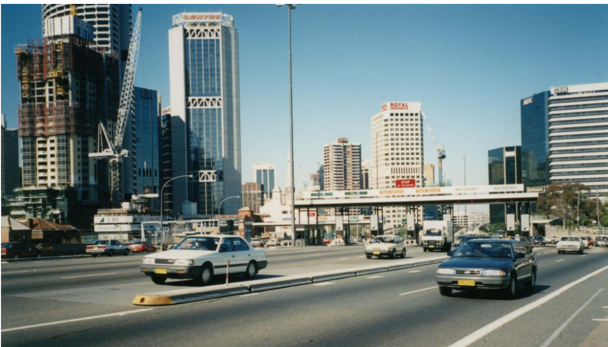
Figure 9.3: Island that can be moved remotely from a traffic management centre
