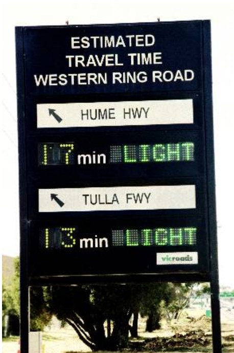
Figure 5.5: Trip condition sign
