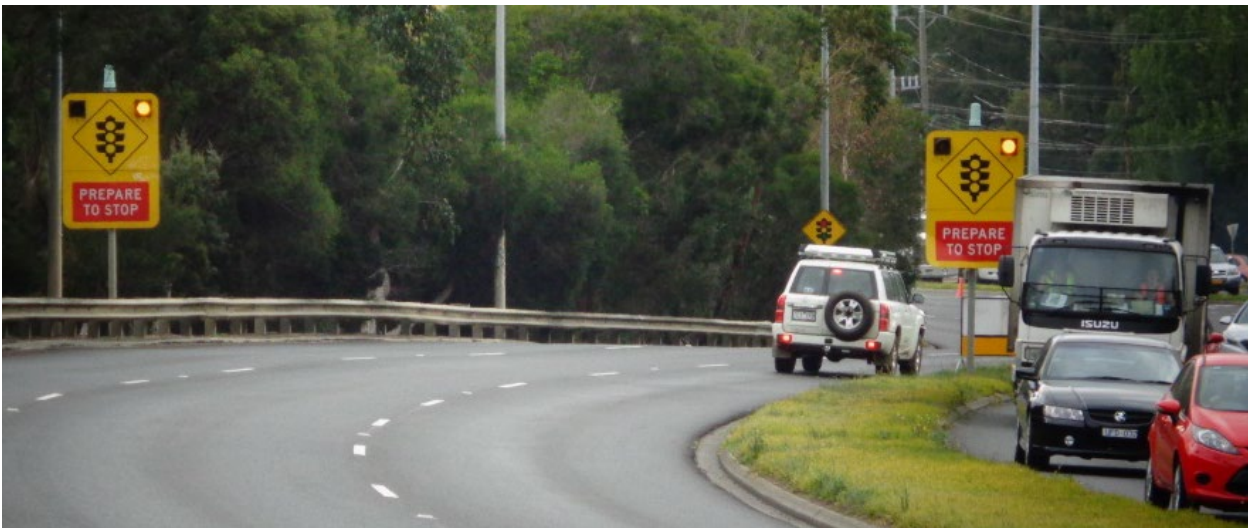
Figure 8.36: Advance warning signal signs in use
