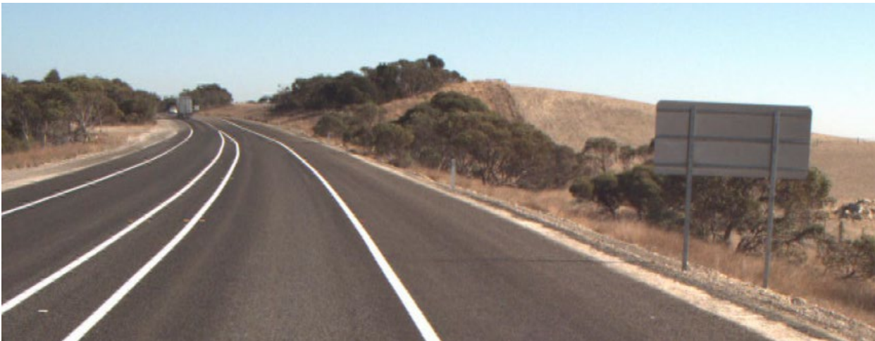
Figure 9.1: Wide centreline treatment example
