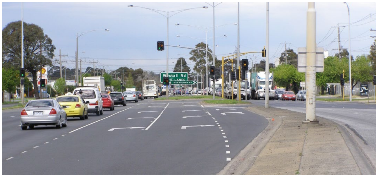
Figure 10.4: Example of a U-turn lane combined with a double right-turn lane
